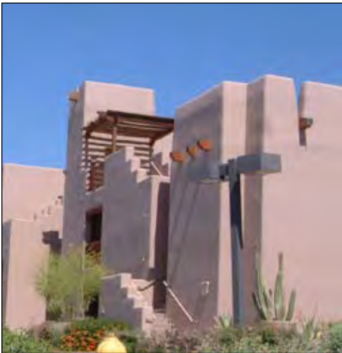
Series 156 Enviro-Crete, a modified waterborne acrylate coating, protects the stucco exterior at the Four Seasons Resort in Scottsdale, AZ.
