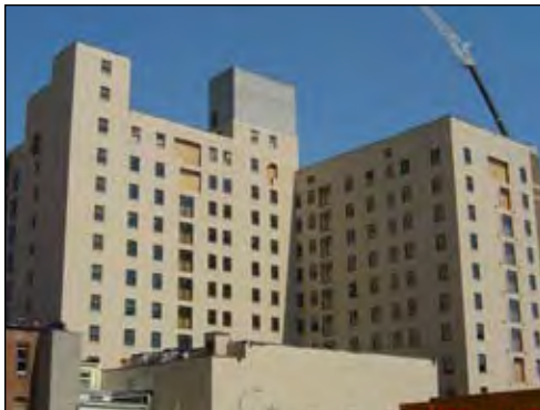
Series 156 EnviroCrete, a breathable coating with excellent elastomeric properties, was chosen to help restore the exterior of the historic Paxton Building in Omaha, NE.
