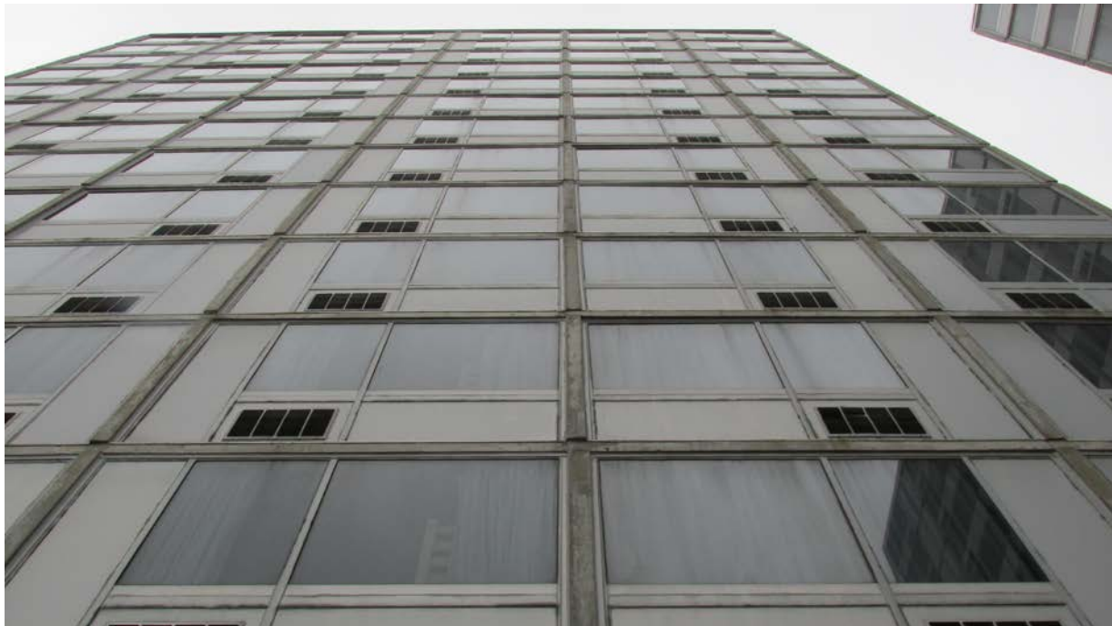
Figure 5 – Existing Tower “D” Façade with Six Bay Entrance Window Wall
