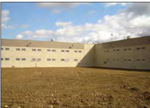
Tnemec coatings were used on both the interior and exterior of the North Branch Correctional Institution in Cumberland, MD.
